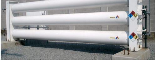
**Fact:** The "Energy Density" is lower than gasoline or diesel fuel, so in order to store the equivalent amount of fuel on the vehicle, we need to compress the gas to a higher pressure.
